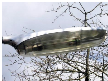
Example of a sodium lamp (not from Cowes) 18
